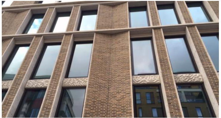
Sasha Holzer Portland Stone Panels on the Façade of 30 Broadwick Street
