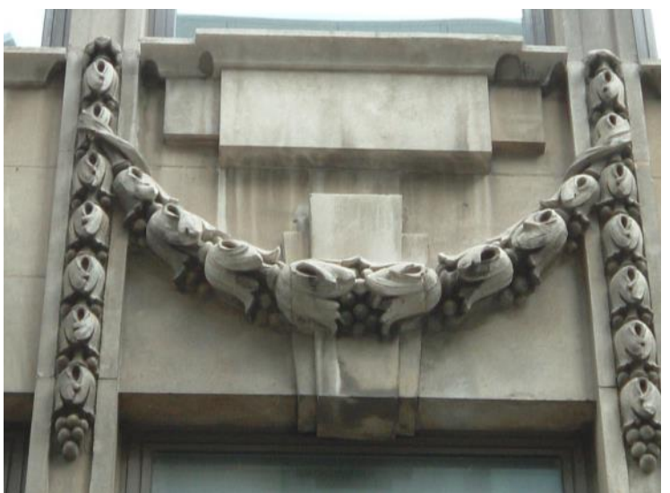
Portland Stone Swag on Fenchurch St Restoration
