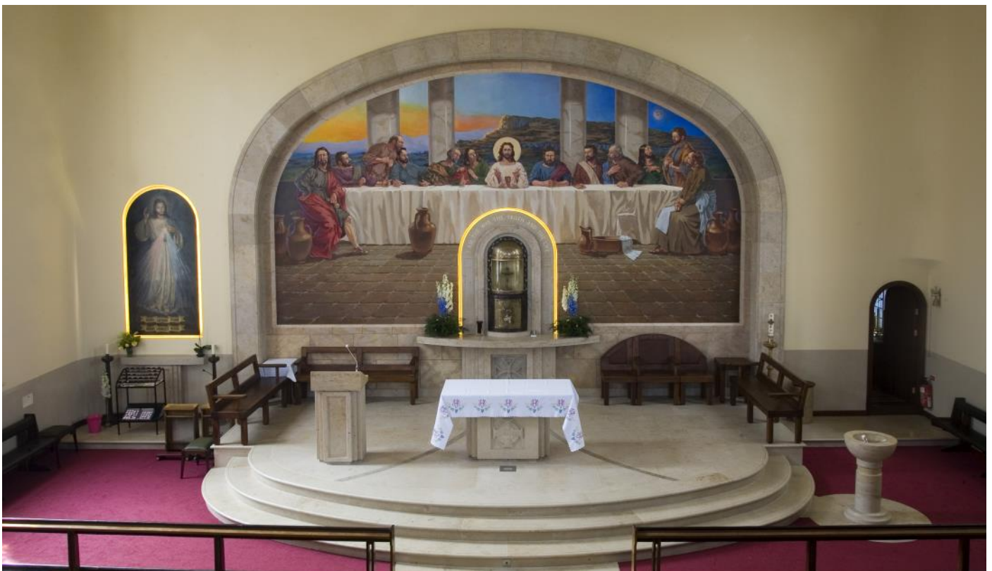
A self-supporting stone arch in St Michael's Church, Birmingham
